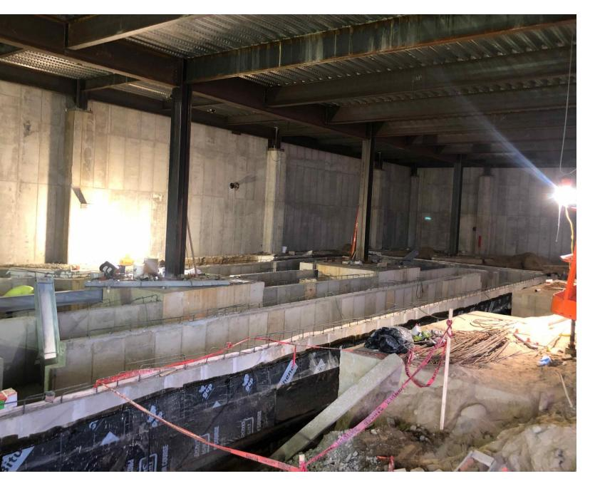
For our two cyclotron systems: controlled flow path that takes the exhaust from the radiopharmacy 100 min to get from the beginning to the end.
